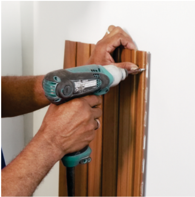
1. Place the Venya Louver on the wall or ceiling
