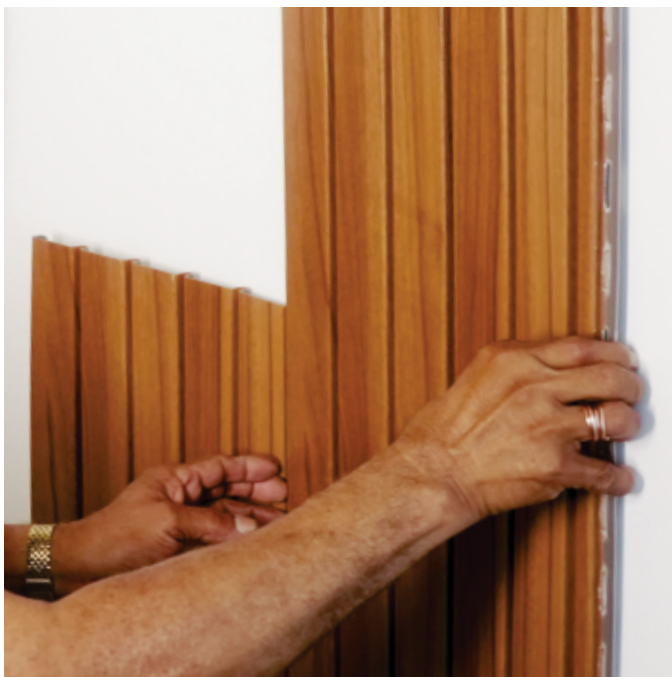
3. Take the second louver and interlock it with the first using 'Rapid-Clad' interlocking technology
